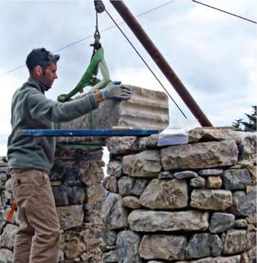
Using the gin-pole to set the lintels.
