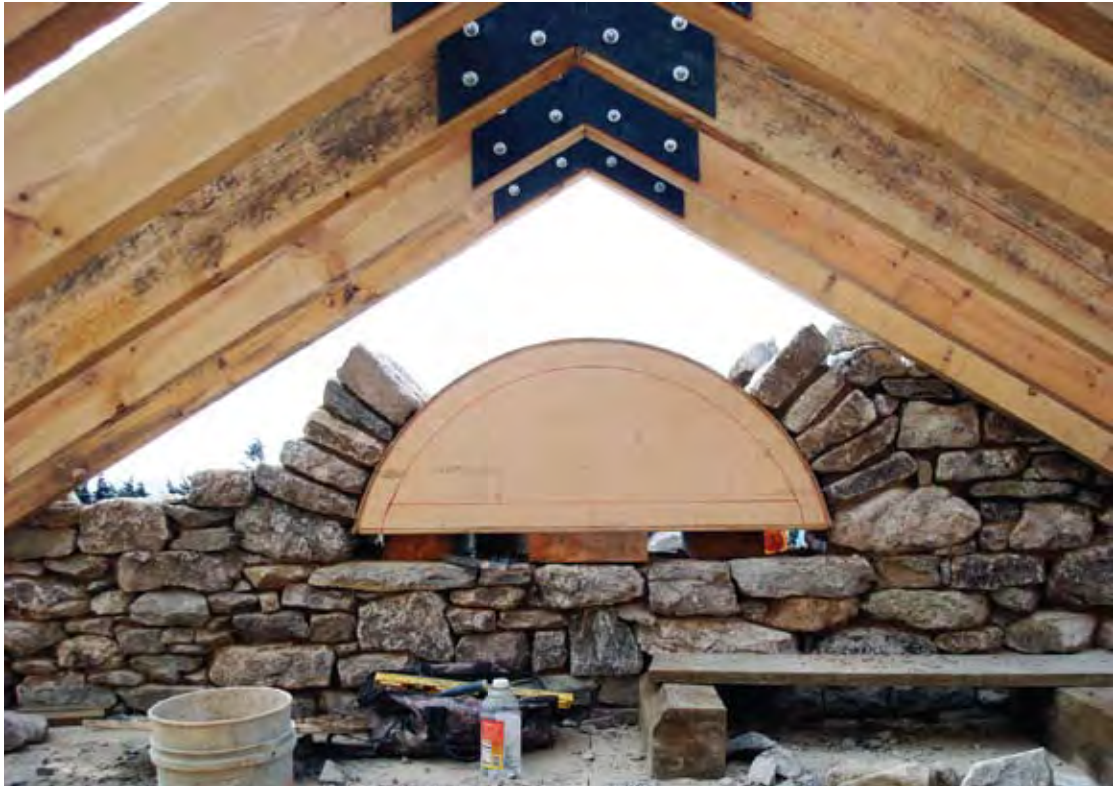
The arch on the cabin face in process. The wall is two feet thick here.
