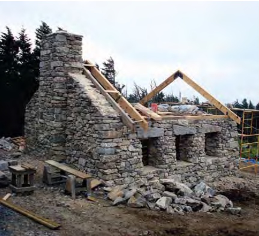
Rear view showing chimney and the first rafters. There are three windows one each side with large granite lintels.
