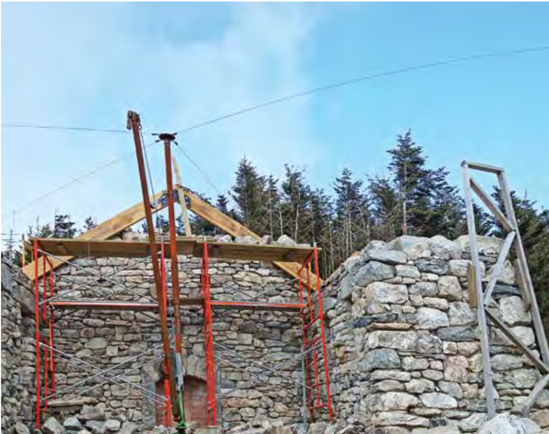
Half a stone cabin. You can see the batter of the walls in the guides we built. The side walls are battered, three feet at the base, two feet at the top.
