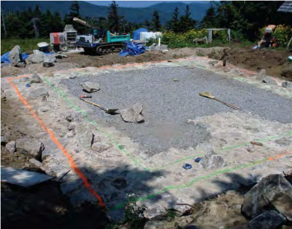
The cabin foundation ready for walls; note protruding stones that will key into the walls.
