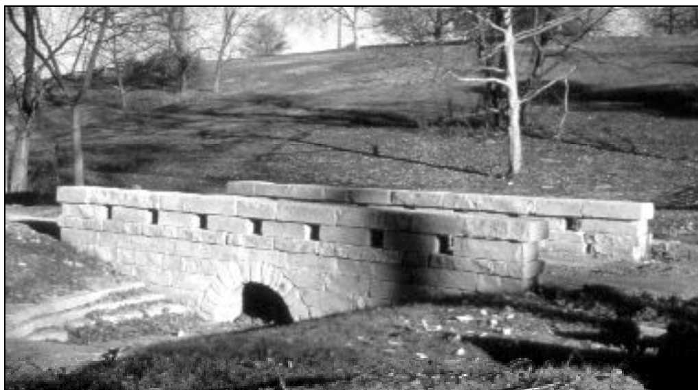
Dry stone bridge and channel lining. Cherokee Park, Louisville KY
