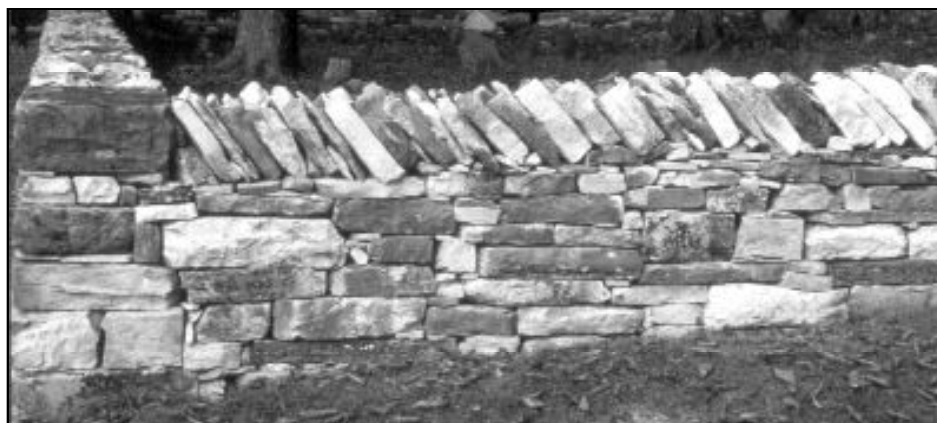
This pre-civil War cemetery wall in Fayette County, Kentucky, was previously in complete ruins. The DSC restored it while training masons in the drystone craft.
