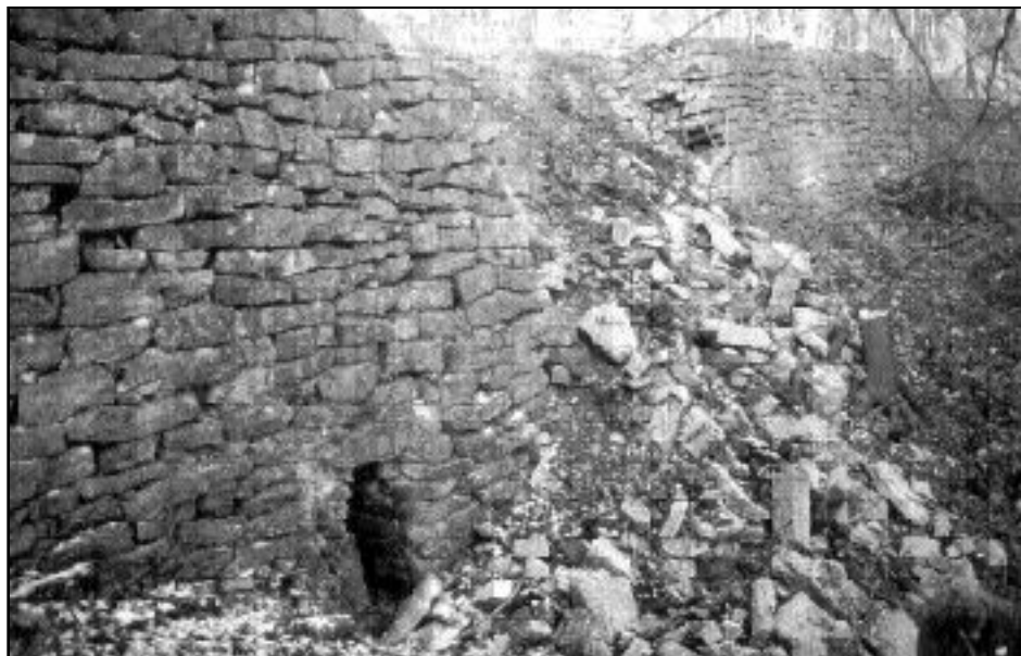
This nineteenth century roadway retaining wall in Louisville's Cherokee Park was built with faults that led to its collapse in 1995.
