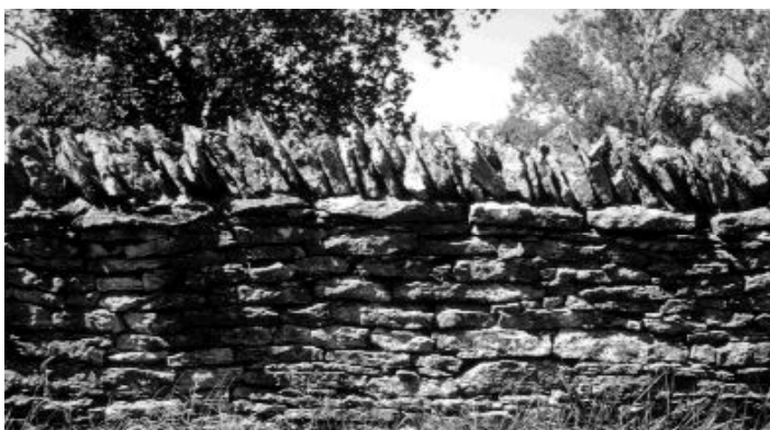
Kentucky rock fence, built of purpose-quarried coursed limestone
