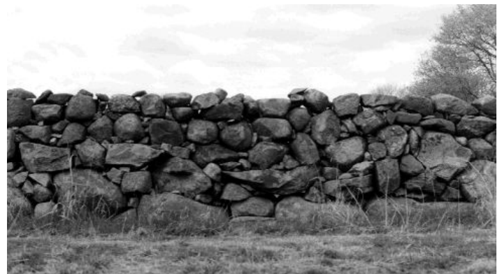
New England stone wall of glacially-rounded granite boulders
