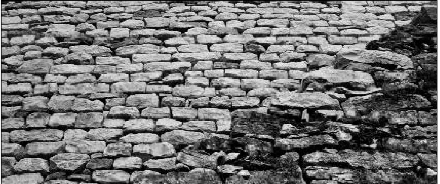
Detail of Schenkenberg vineyard wall. The new wall was built behind the old and a staircase was created.
