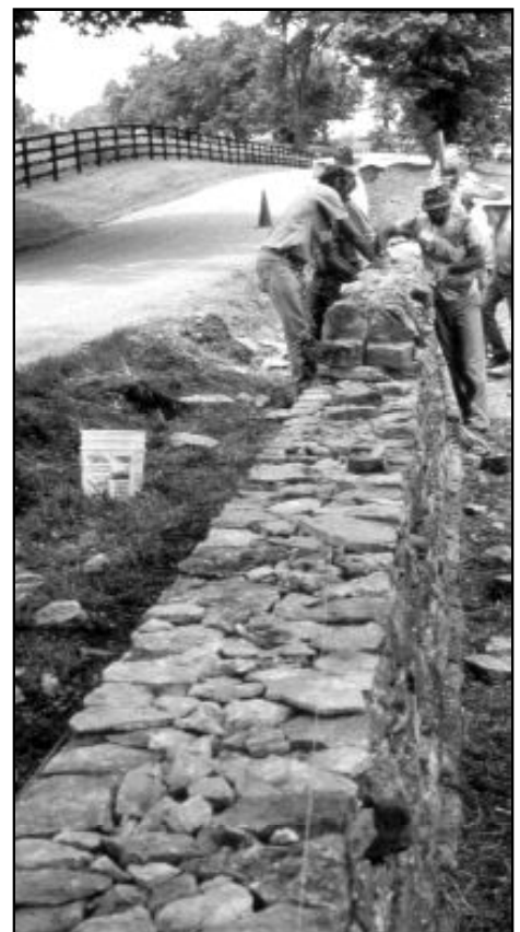
DSC training projects include relocating historic rock fences affected by roadway projects.
