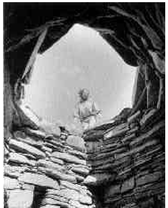
John O’Leary at work while corbelling ‘Shelter of the Bay’
