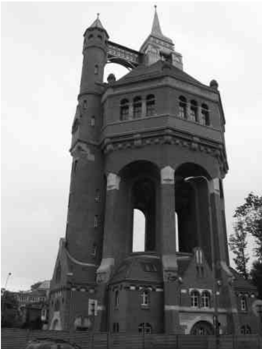
This water tower, constructed following devastating flooding in 1903, is a good example of how brick work can be effectively combined with stone. While carved stone is used sparingly here, imagine how different this building would look without it.
