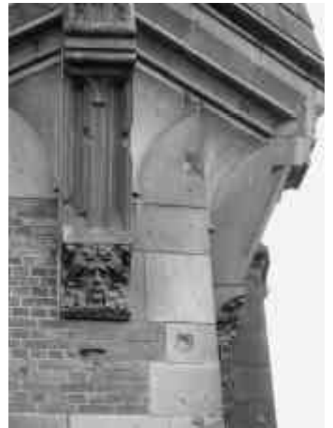
This water tower, constructed following devastating flooding in 1903, is a good example of how brick work can be effectively combined with stone. While carved stone is used sparingly here, imagine how different this building would look without it.
