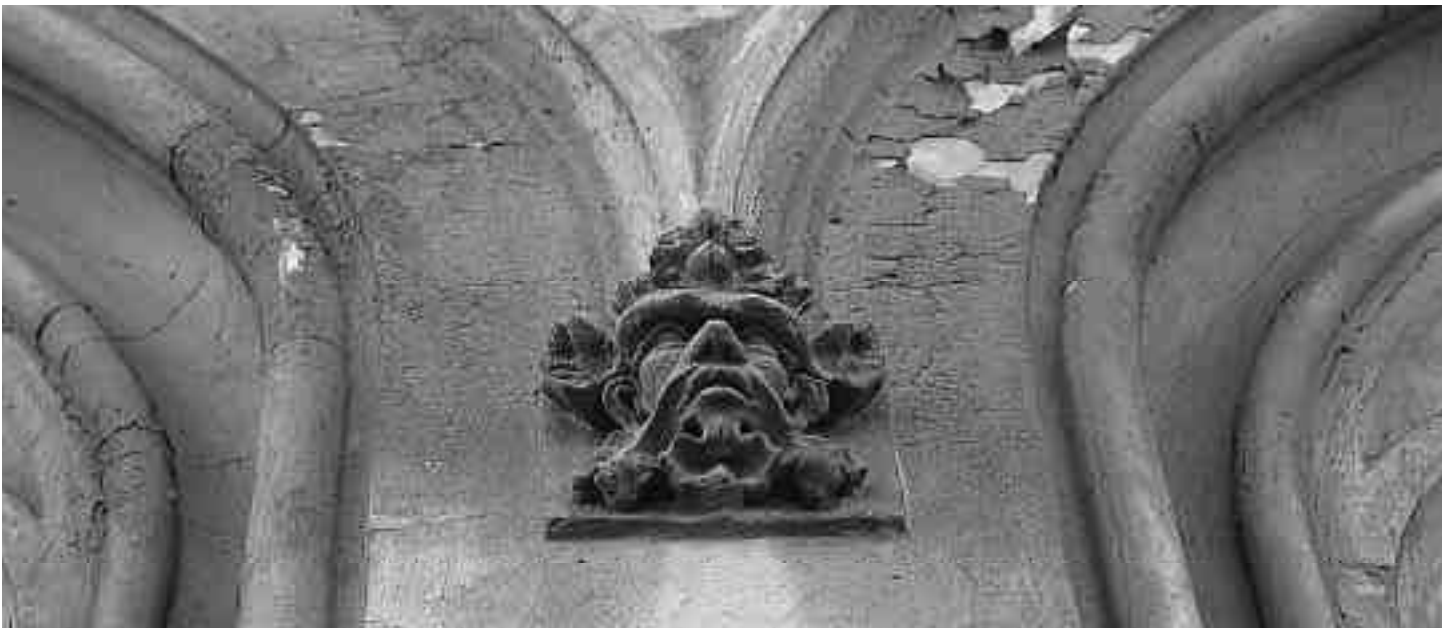
This green man on the facade of the Exchange Building serves as a springing stone for two arches. (Wroclaw, Poland)
