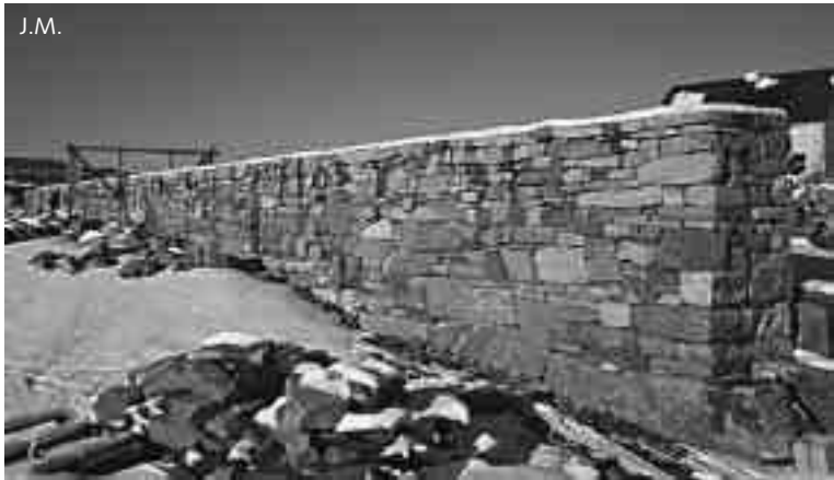
Wall, South Kent, CT
