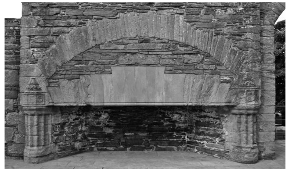
The arched opening of the fire-place is fifteen feet wide; note the way the voussoirs (arch stones) are shaped. The flare at the upper end serves to lock them into place. Still, it must have failed at some point, but the arch of discharge in the fabric of the wall above it performed as intended and held the weight of the upper masonry so that the arch could be replaced.
