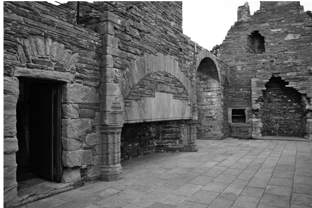
The arched opening of the fire-place is fifteen feet wide; note the way the voussoirs (arch stones) are shaped. The flare at the upper end serves to lock them into place. Still, it must have failed at some point, but the arch of discharge in the fabric of the wall above it performed as intended and held the weight of the upper masonry so that the arch could be replaced.
