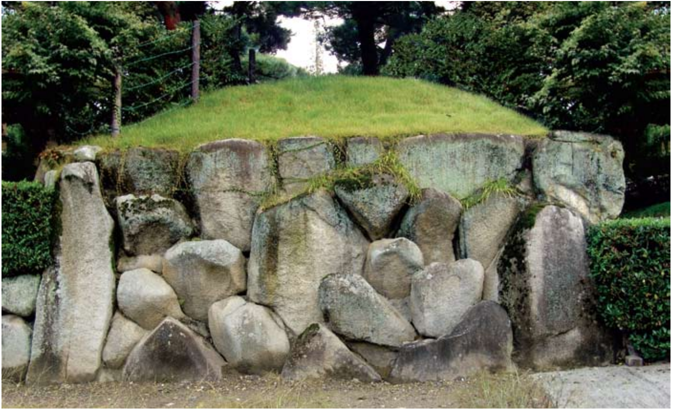
above: Japanese basalt boulder retaining 'wall.' photo: Carl Johannsen
