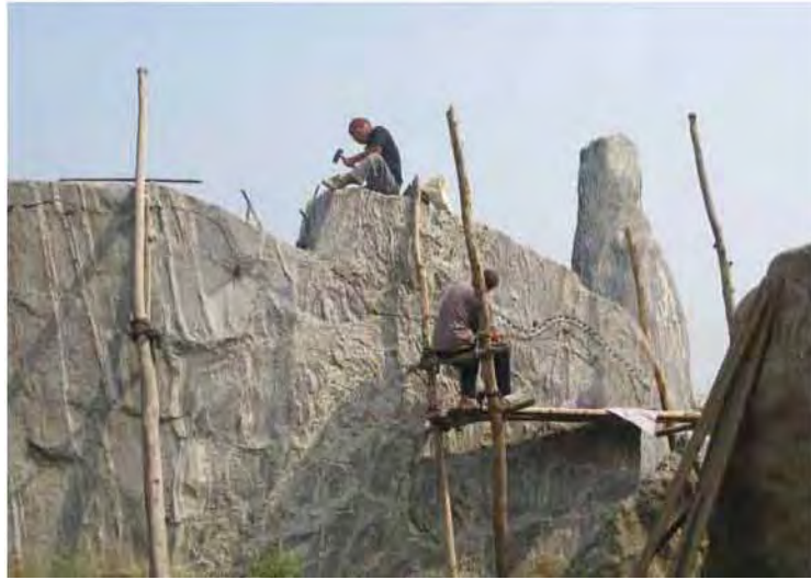
left: Altering the profile of a natural river boulder, Hebei, China.
