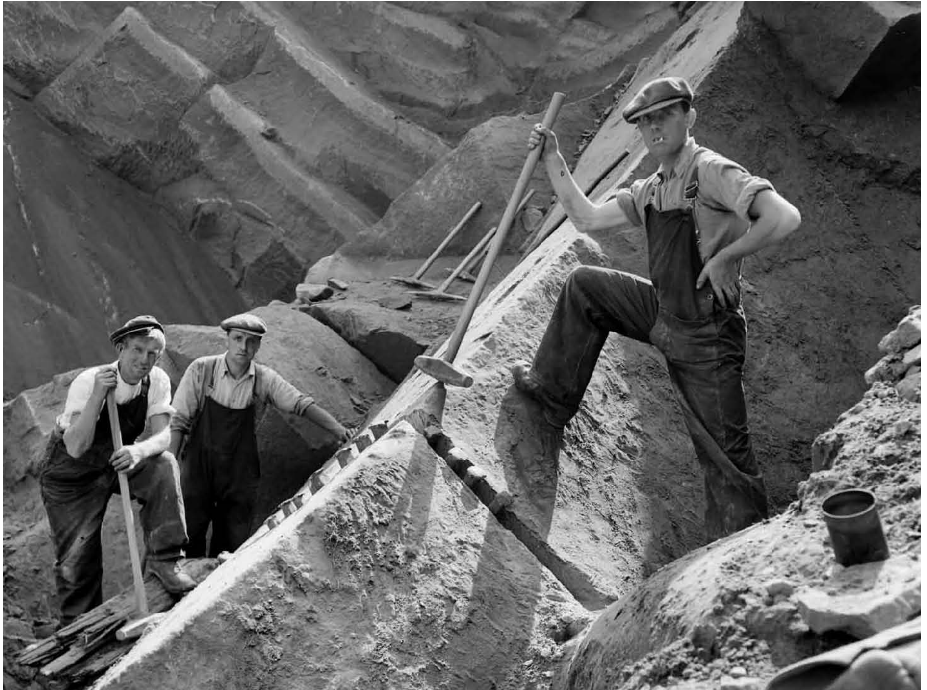
Quarrymen splitting sandstone by the chisel and wedge method. Corncockle quarry, Lochmaben, Scotland, 1937.
