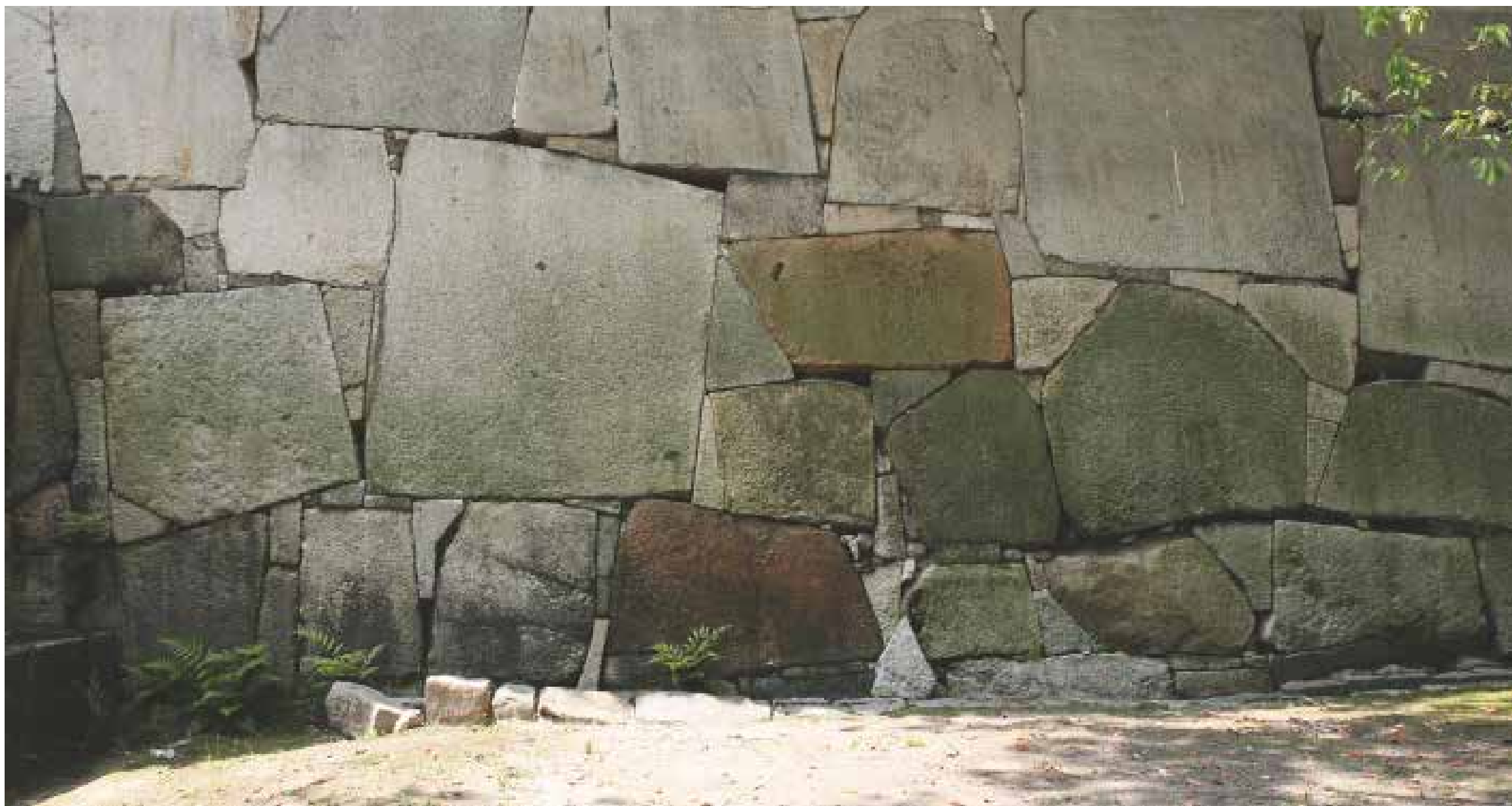
Wall, skillfully constructed using recycled fragments, Osaka Castle precincts, Japan. photo: T L
