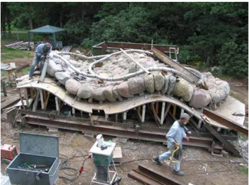
Fixing the top and the bottom steel frames together, preparing to lift off.
