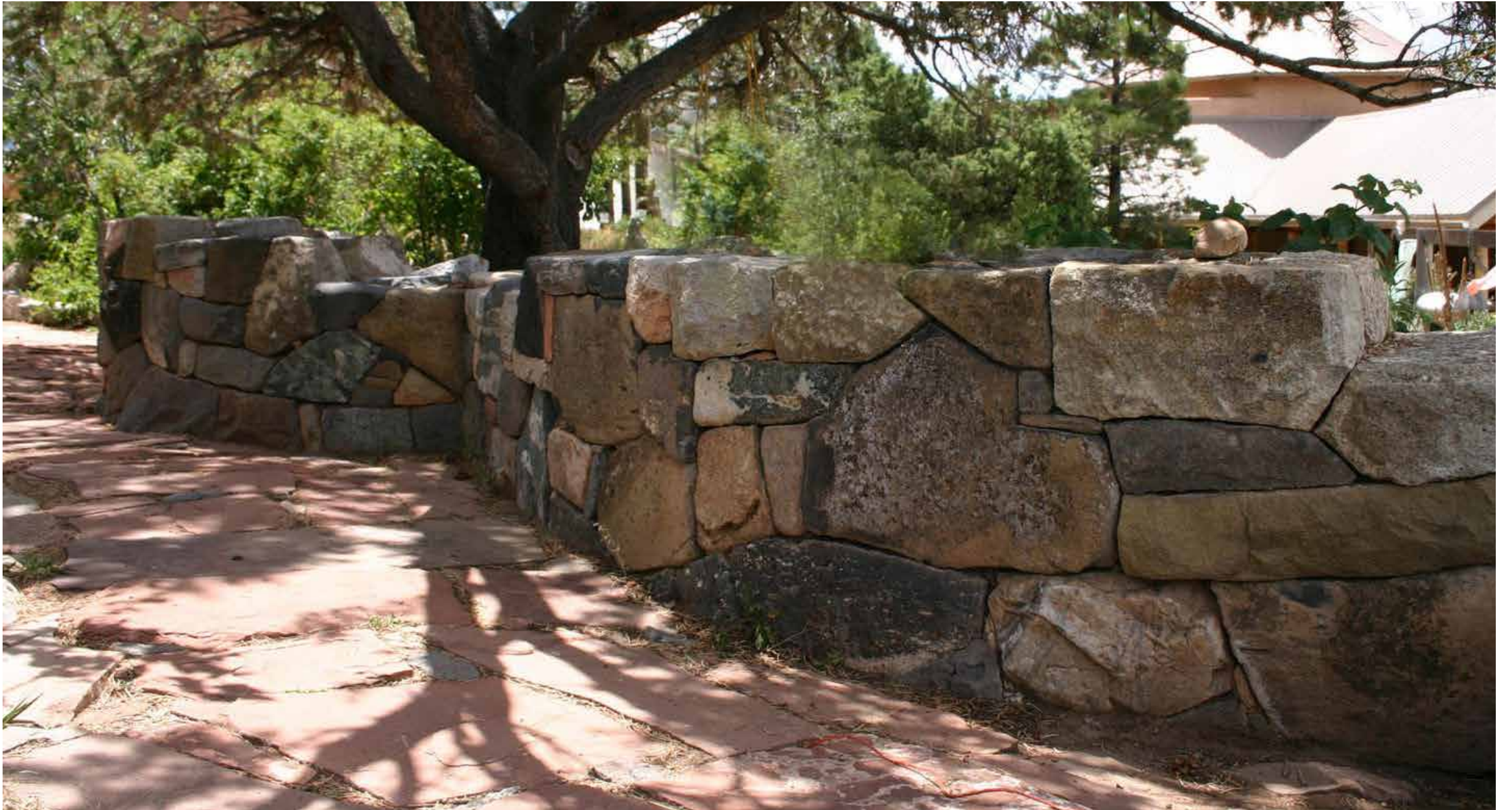
Dry stone wall, Stone Foundation workshop project, 1986, Lama Foundation, Northern New Mexico. photo (2004): T L
