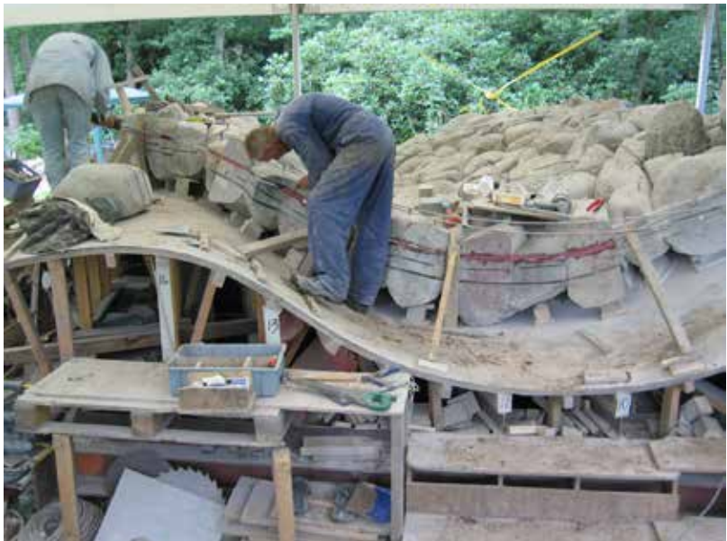
Fixing post-tension stainless steel cable into the penultimate layer.
