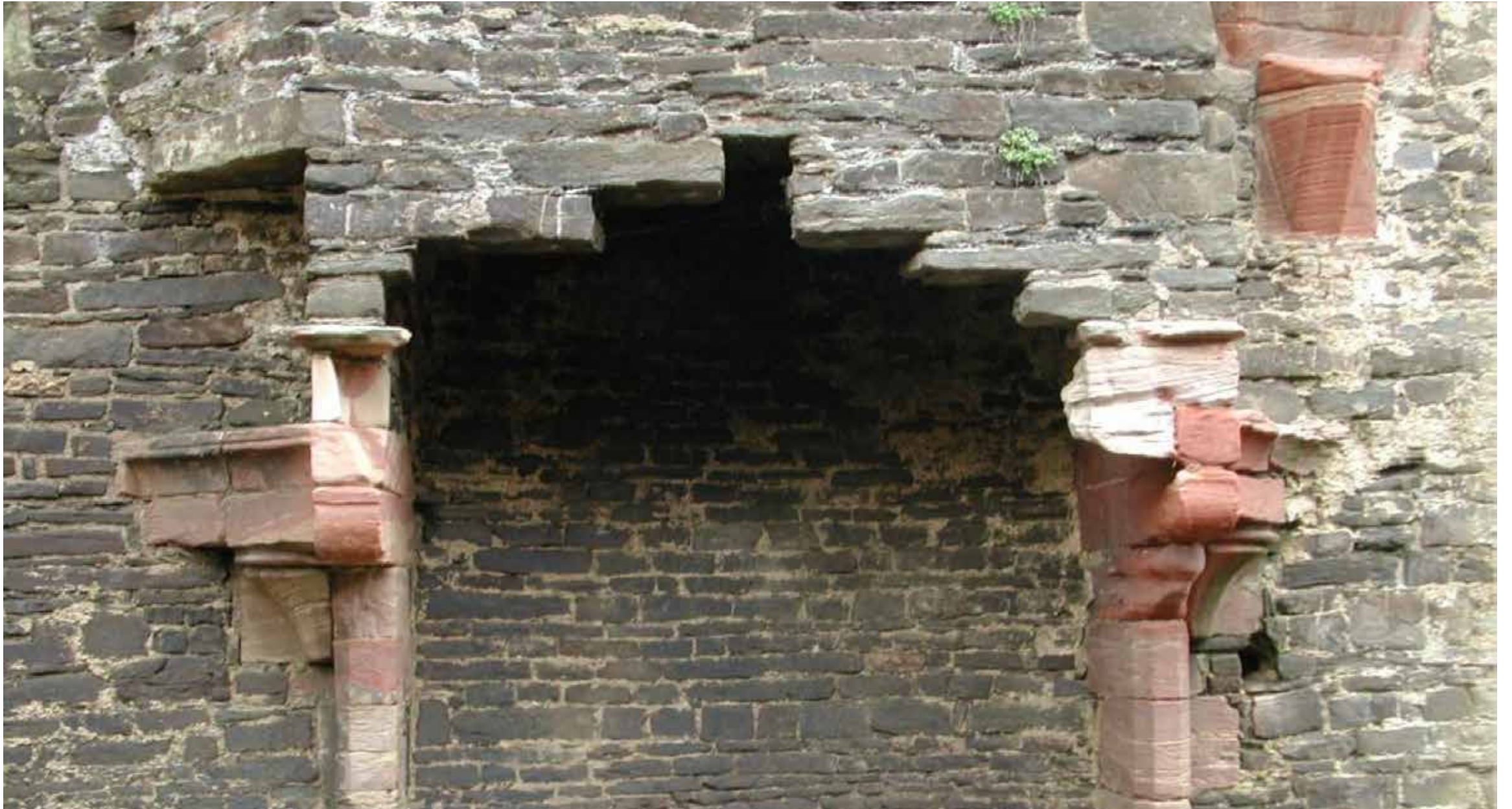
Conwy Castle, Gwynedd, North Wales. The lintel over the opening of this fireplace has failed, but the bonded stonework over it has formed a structural, corbeled 'relieving arch' that serves to support the mass of masonry above. photo: ?
