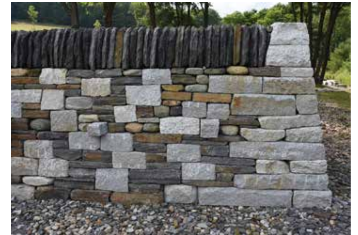
above: Dry-stone wall, certification project by Jared Flynn
