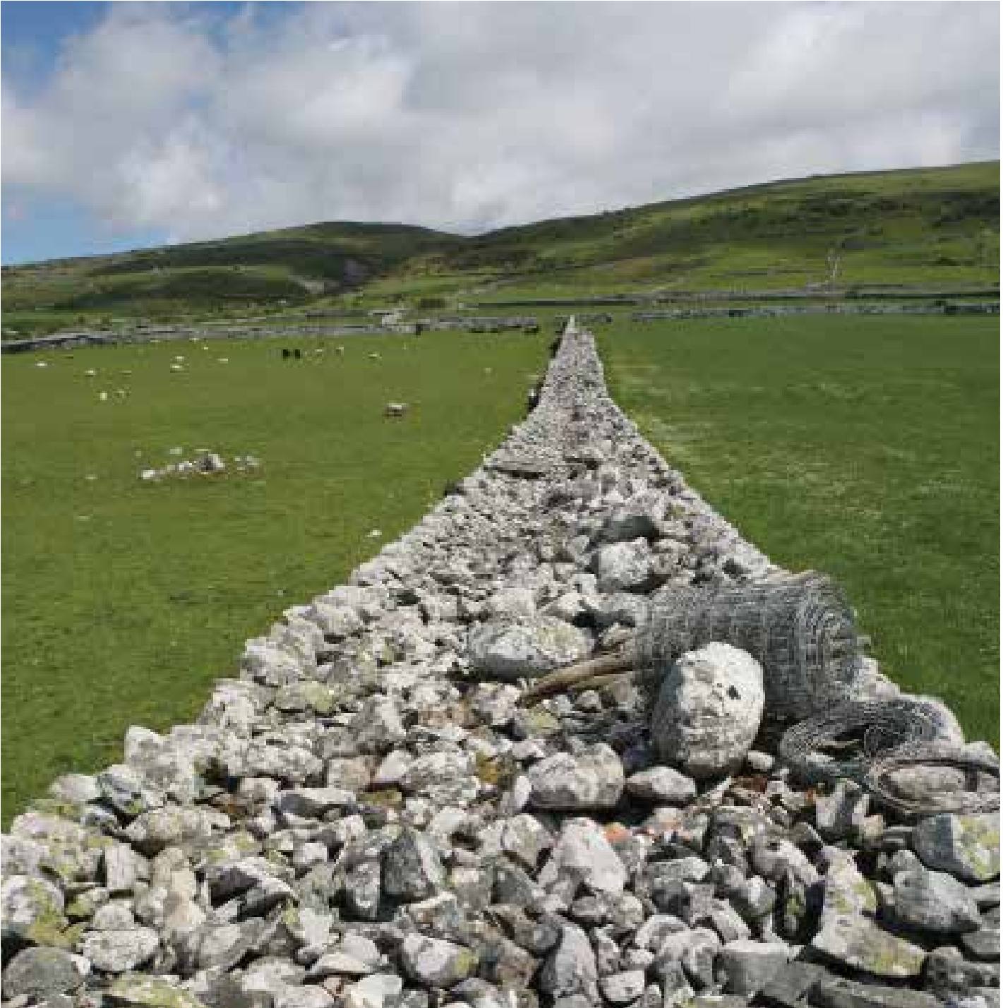
A megalithic CONSUMPTION WALL at Egryn near Harlech. Consumption walls can be found scattered throughout the UK, commonplace in some areas, only occasionally in others. Their purpose is, as their name implies, to literally consume the stone continually being cleared from the adjacent fields. This wall near Harlech at about 8 feet across is possibly the widest in north Wales, but it pales in comparison to the Kingswell dyke near Aberdeen in Scotland, at 27 feet, the widest in the UK.
