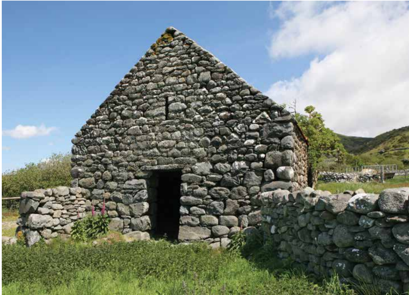
DRY-STONE COW BARN at Egryn near Harlech. An exceptionally well-built structure, this face features the entryway, a ventilation slit and an enclosure in front framed by dry-stone walls. Date uncertain, but the construction style is compatible with the 18th century.
