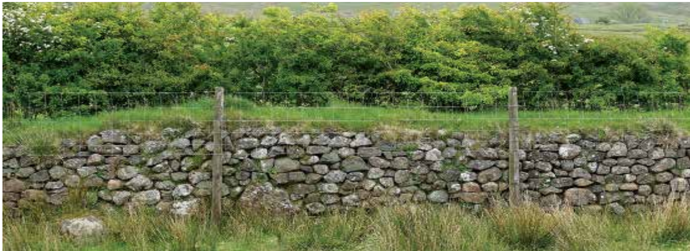
top: Roadside field wall near Dunnerdale, Duddon Valley. This style of coping with slates between rounded field stone occurs in a number of locations scattered around Cumbria. above: Stone-faced earth bank. Common in Cornwall and Wales (known as clawdd walls there) but a rarity in Cumbria. Not really
