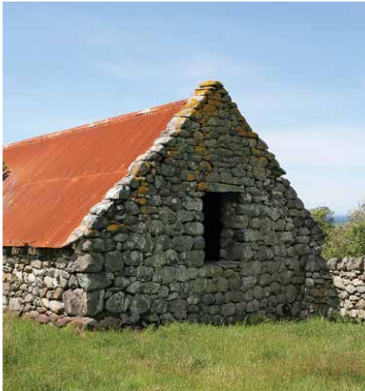
DRY-STONE COW BARN at Egryn near Harlech. An exceptionally well-built structure, this face features the entryway, a ventilation slit and an enclosure in front framed by dry-stone walls. Date uncertain, but the construction style is compatible with the 18th century.
