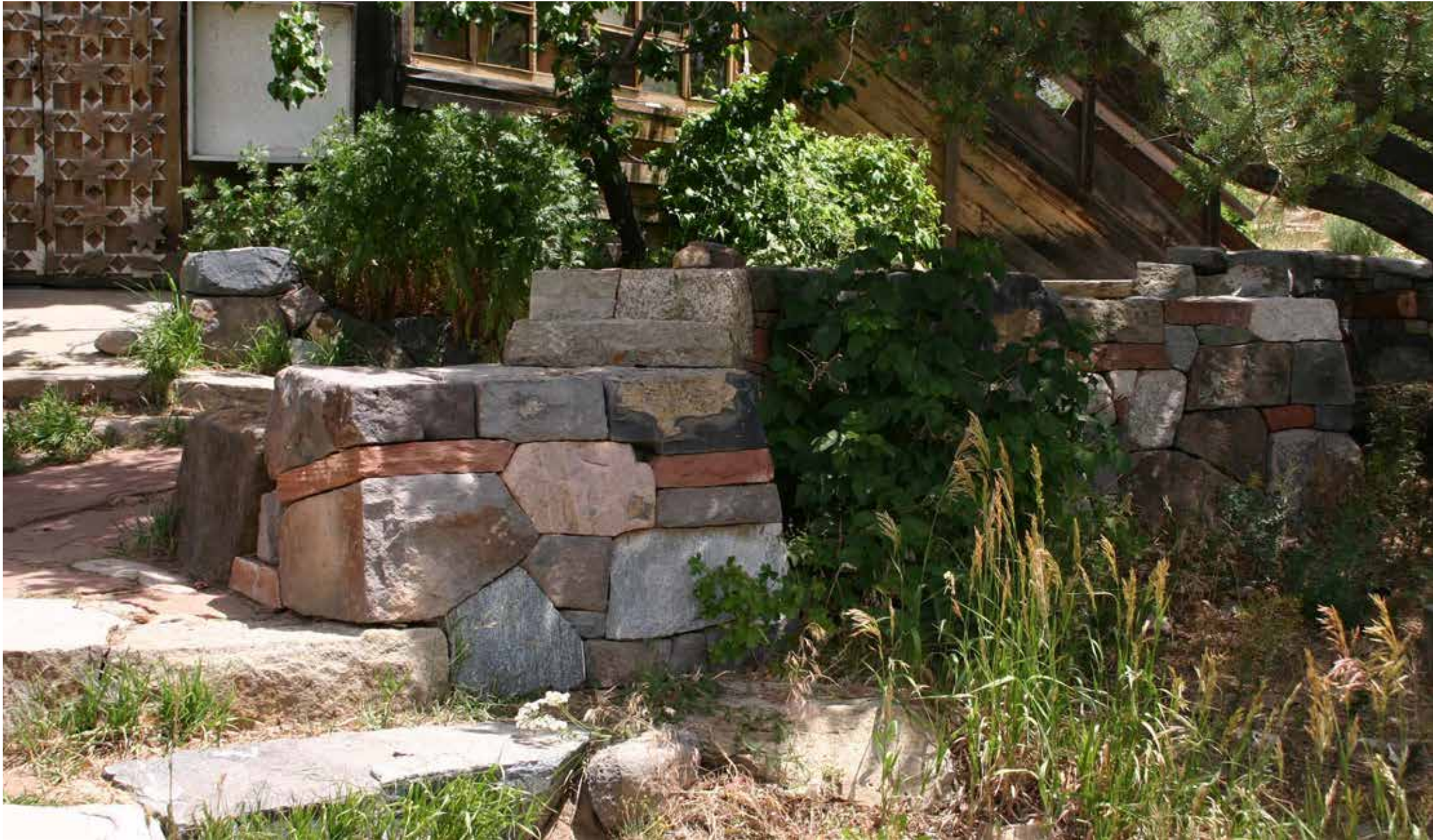
Dry stone wall, Stone Foundation workshop project, 1986, Lama Foundation, Northern New Mexico. photo (2004): T L
