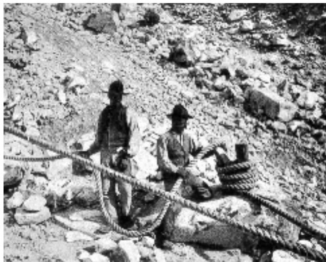
below: A 'socket' carved in a rock outcropping into which the posts, are placed. From this photo it seems that taller posts were placed in the deeper center hole and shorter posts were hammered into place around those to tighten the 'bundle.' Obviously steel cables were employed here.
