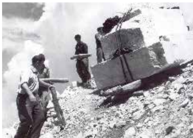
above: At Carrara, a loaded sledge (lizzatura) being lowered down a steep slope. The men are taking small wooden beams from behind the sledge and placing them in front of it. The beams were smeared with soap to facilitate the passage of the sledge runners.
